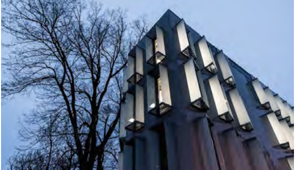
PLATOU CLARKSON OFFICES BUILDING - OSLO (NORWAY)
