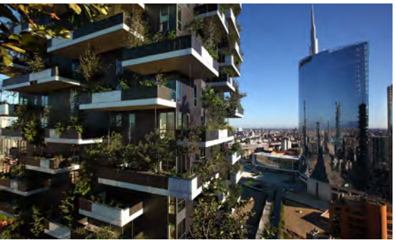
BOSCO VERTICALE PRIVATE APARTMENT RESIDENTIAL - MILANO (ITALY)
