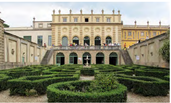
VILLA SALVIATI BUILDING - FIRENZE (ITALY)
