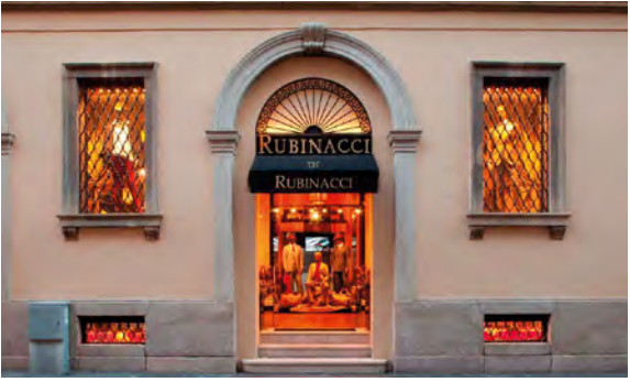
ATELIER RUBINACCI BUILDING - MILANO (ITALY)
