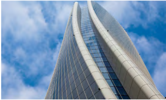
TORRE HADID OFFICES BUILDING - MILANO (ITALY)
