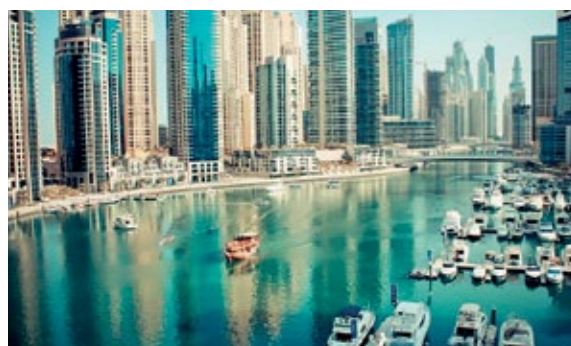
IRIS BLUE TOWER DUBAI - (UNITED ARAB EMIRATES)
