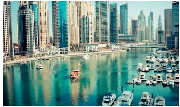
IRIS BLUE TOWER DUBAI - (UNITED ARAB EMIRATES)
